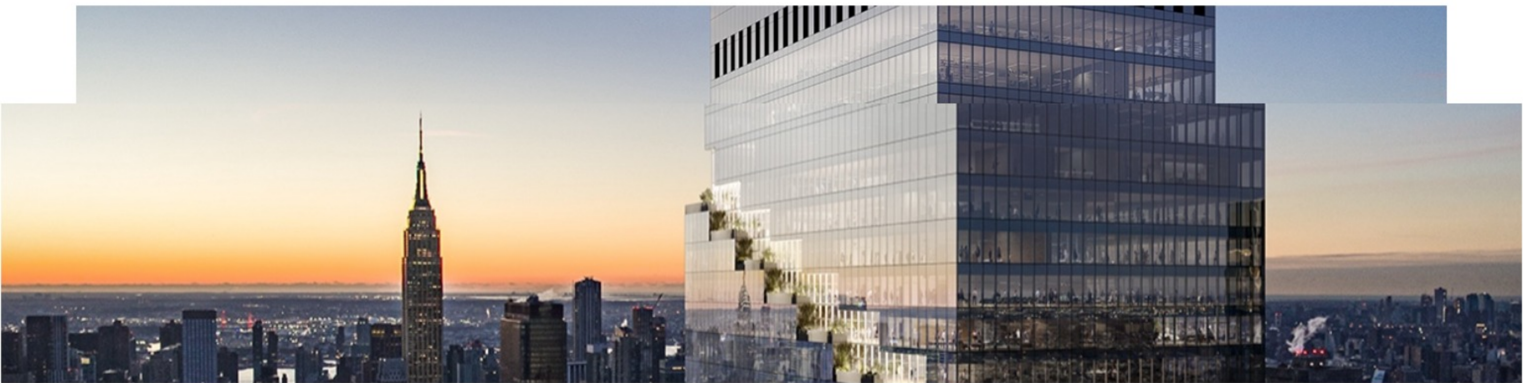
When he was working on The Spiral office tower in Manhattan’s Hudson Yards, Smilow used steel to help overcome a daunting set of engineering challenges. Image by Binyan Studios.
